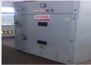
Using electrical power compensation device
