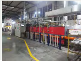
Revamping of electric heating equipment
