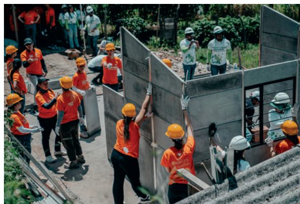
Dream Builders program: construction of homes in Colombia
