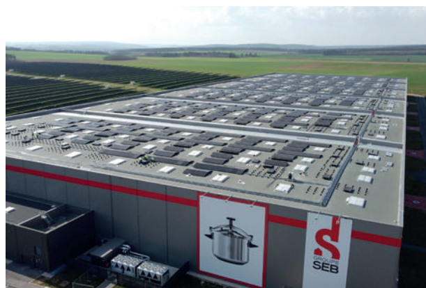
Installation of a photovoltaic power plant in Til-Chatêl
